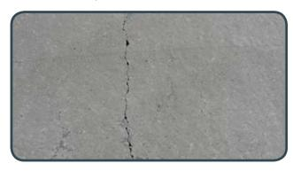
Despite adopting good design, detailing and construction practices, such as control joints and reniforcing mesh, to minimise the risk of cracking, there will be situations where cracks may occur as a result of movements in concrete due to changes in its moisture content and temperature.
