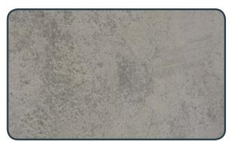
A particularly severe type of discolouration that may appear as the concrete dries out is 'pinto'. The possible causes of pinto are many and varied, ranging from hard-troweling that densifies and darkens the surface through to moisture transfer from adjacent soil.
