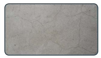
Cracks wider than 1mm should be assessed on an individual basis in terms of possible effects on durability and performance requirements and, depending on the surface texture and finish, also on aesthetic requirements.
