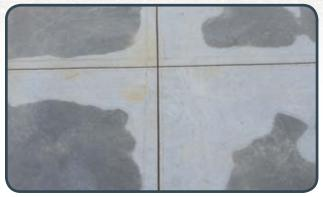
Letting the concrete weather may reduce the contrast in colour but does not always produce satisfactory results. Various proprietary applications are also available to mitigate the appearance of pinto.
